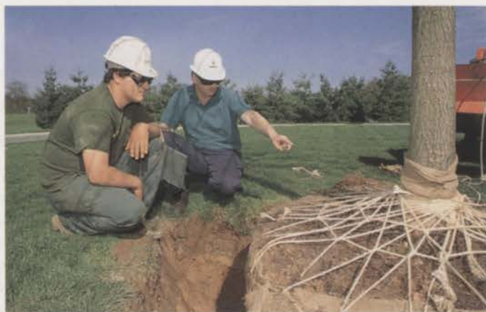
Ensuring that trees and shrubs are properly set within the right size hole is key to successful plantings. Photo: Davey Tree
