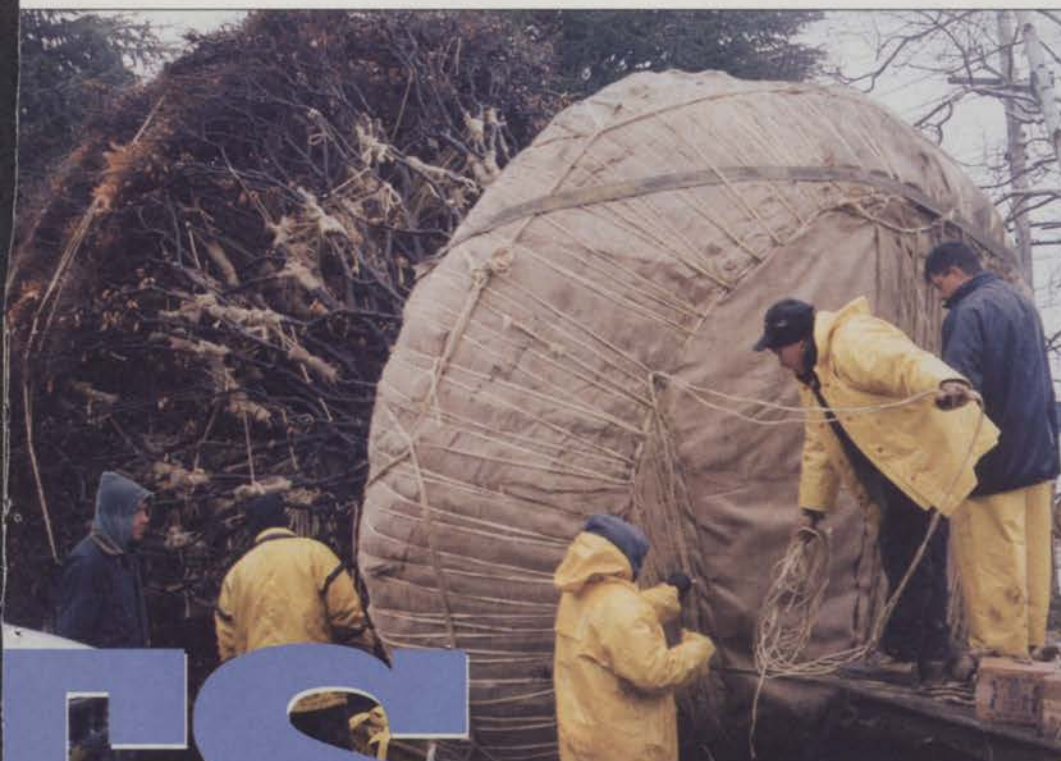
Prior to the transport of a large tree specimen, contractors must prepare the rootball for the journey. This involves careful attention to the method of removal, whether using a tree spade or cutting roots by hand, and a look at the moisture, soil and general health requirements of the tree's root system. Top photo: Chapel Valley Landscape Company, Lower photo: Marders
