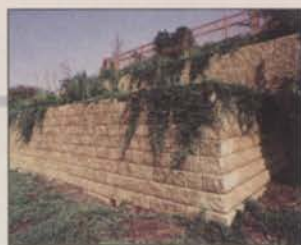
Photo: Anchor Walls.
