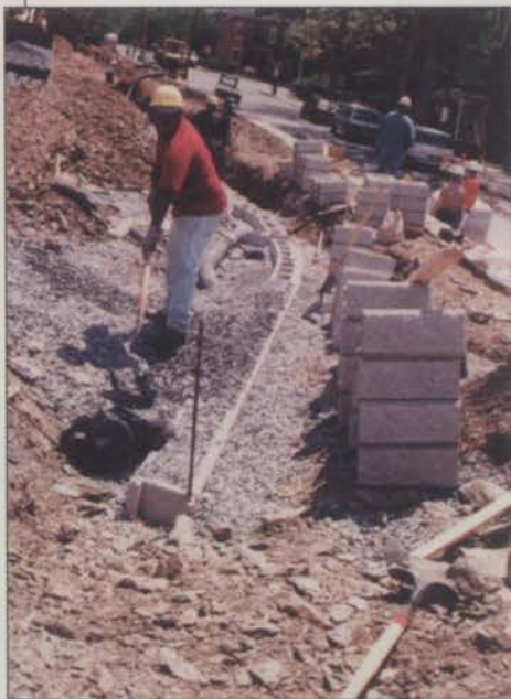
A solid, properly engineered foundation is critical to the success of a retaining wall. Photo: Anchor Walls.
