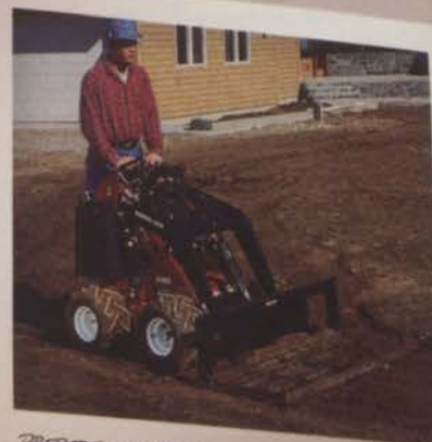
PREPARE THE PATIO SUB-GRADE USING THE LEVELER. ALSO USE IT TO FINISH THE FINAL GRADE.
