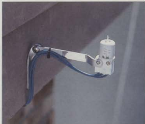
Rain sensors are only effective if installed properly. They should extend out from a house, for example – not mounted underneath a gutter or eave.
