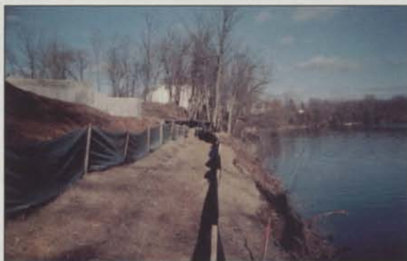
Riverbanks can be protected against erosion with a silt fence and straw blanket (above) or with coconut logs planted with aquatic vegetation (below). Photos: Designs By Nature.
