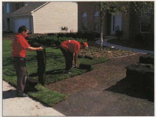
Before sod is installed, contractors should give special consideration to the layout of the land. Photos: Turfgrass Producers International (top) and Delta Bluegrass Co. (bottom).
