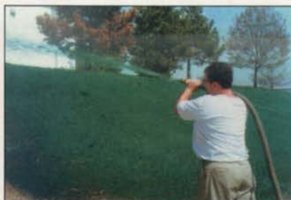
Contractors can add a material similar to glue called tackifier to their hydroseeding mixes so it will stick, particularly in hilly or steep areas where making sure the seed binds to the soil so it has a chance to germinate is important. Photos: Finn Corp.
