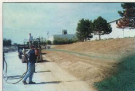
Contractors can add a material similar to glue called tackifier to their hydroseeding mixes so it will stick, particularly in hilly or steep areas where making sure the seed binds to the soil so it has a chance to germinate is important. Photos: Finn Corp.
