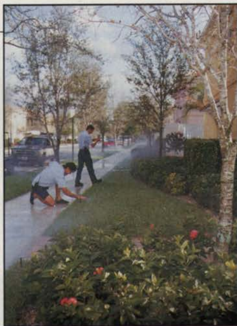
Pop-up sprayheads or rotors should always be selected to rise above the immediate turf or shrubs. Photo: Peter Hughes
