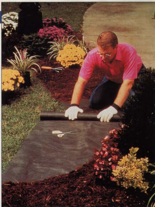
One function landscape fabric serves is weed control. When it is used in this capacity, it should separate the mulch from the soil and limit the maintenance required for beds. Photo: Reemay
