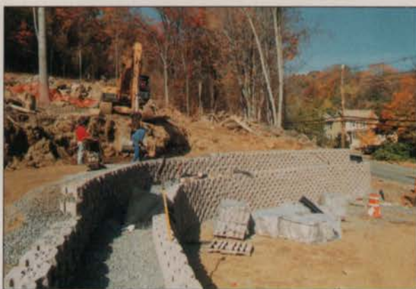
Installing retaining walls of all shapes and sizes requires careful consideration of the type of soil held back by the wall for long-term stability. Photo: Keystone
