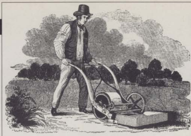
A representation of Budding's 1830 gear-driven mower equipped with a cutting cylinder that rotated very close to the lawn's surface. Photo: Textron Turfcare & Specialty Products
