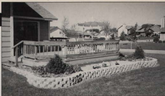
Smaller, modular concrete walls (left) can easily create more usable space as part of the landscape. Photo: Keystone
