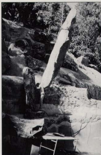
Boulders, weighing as much as 15 tons, were positioned over the house by a crane operator relying solely on radio contact to "see." Credit: Bertotti Landscaping
