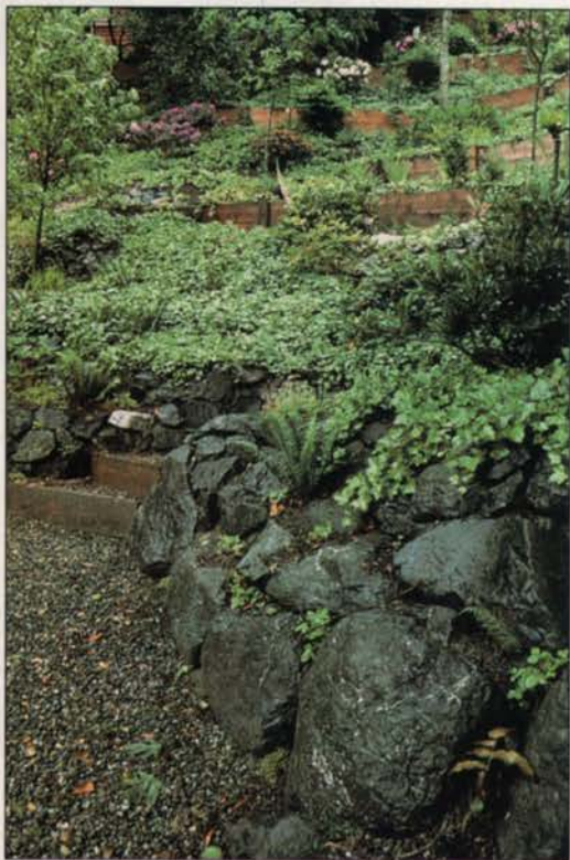
Topsoil was kept on the 35-foot sheer cliff with three-foot retaining walls and erosion netting. Credits: Hendrikus Schraven Landscape Construction & Design
