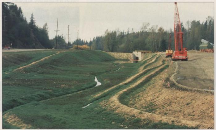
Several swales in this erosion project divert water, including one that catches highway runoff. Photo credit: Weyerhaeuser
