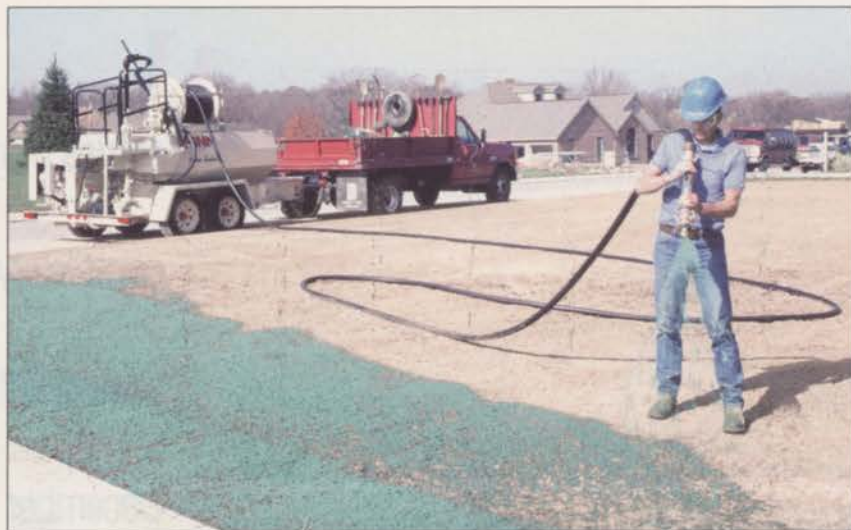
Speed and cost savings are two features of hydraulic seeding. Credit: Finn Corp.
