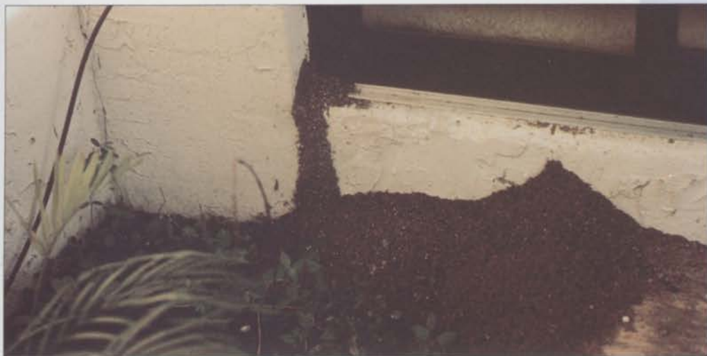
Fire ants may enter structures while foraging for food.
