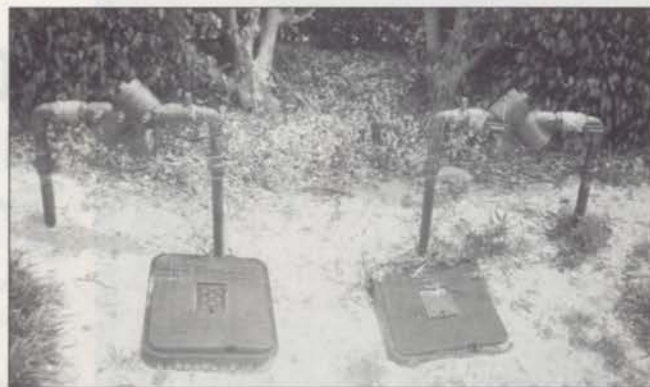
Different backflow preventer assemblies can protect against backsiphonage or backpressure, depending on the system's configuration. Photo credit: Wilkins Regulator, Zurn Industries (left) and Febco (right).
