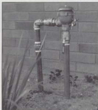
Different backflow preventer assemblies can protect against backsiphonage or backpressure, depending on the system's configuration. Photo credit: Wilkins Regulator, Zurn Industries (left) and Febco (right).
