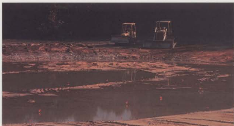
Testing the degree of moisture at each grade level at the Piney Orchard mitigation pond in Maryland helped determine grading requirements and proper plant selection for each level. Photos: Ruppert Landscape Co. Inc.
