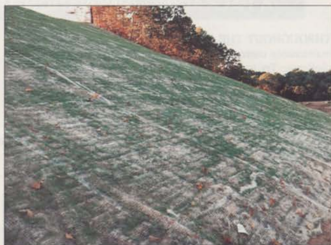
Super Grow from Phillips 66 was used to stabilize this property in New England. Despite two inches of rain after application, the grass turned out fine. Photos: Blunk's Wholesale Supply.
