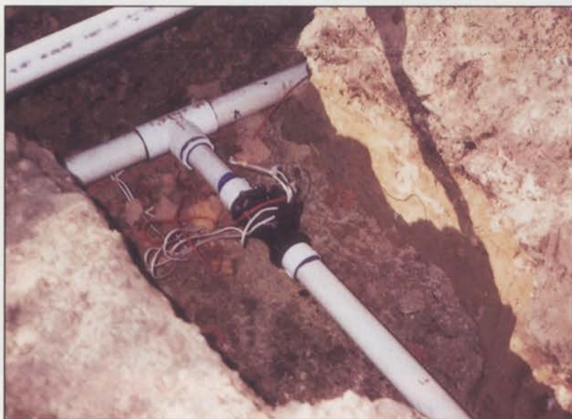
Install valve wiring with plenty of slack for servicing the valve. Photo: Eastern Irrigation Consultants.
