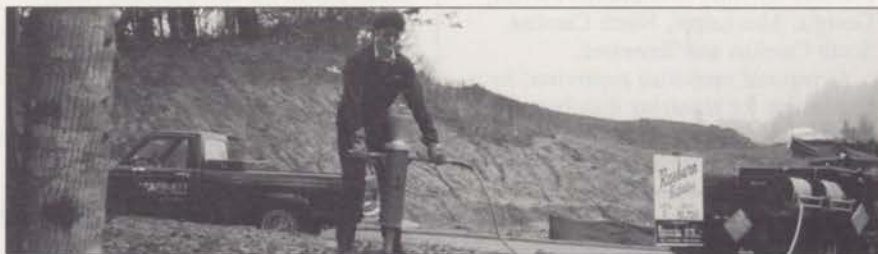
To relieve compaction, holes are drilled every four to six feet.
