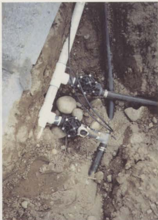
Two valve manifold with a PVC mainline and polyethylene laterals.
