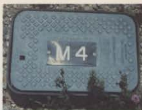
This electric remote control valve access box, with attached identifying laminated plastic tag, identifies the RCV to a particular controller and control station.
