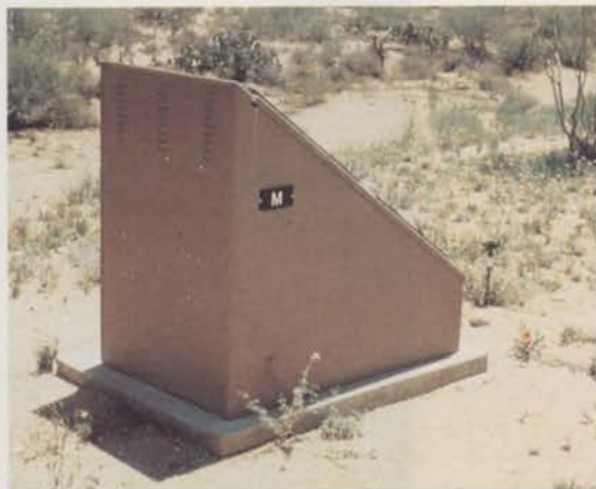
This cabinet contains a solar-powered irrigation controller. Note the identifying laminated plastic tag attached to the cabinet.
