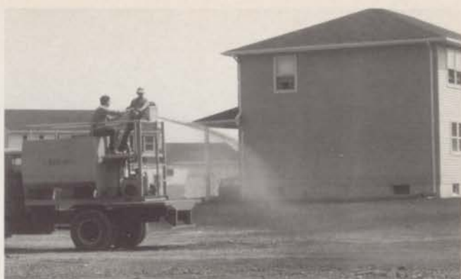
Hydroseeding applies seed, fertilizer and mulch. Photo: Reinco.
