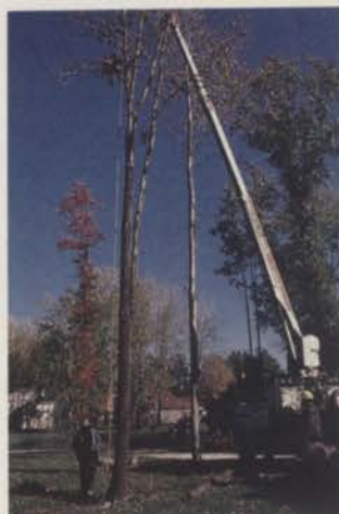
Employees from Ajax Tree and Landscape Service perform brick work (above) and tree pruning below. Photos: Mickey Jones.
