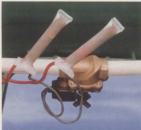
A typical valve from an irrigation system showing the low voltage wiring and splices. Photo: Paige Electric.
