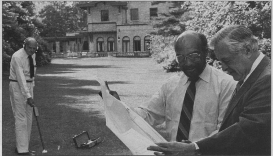
The search continues for 1,300 sprinkler heads on the Henry Ford Estate in Dearborn, Mich.
