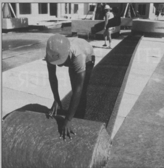
Enkadrain filtering fabric acts as drainage medium.
