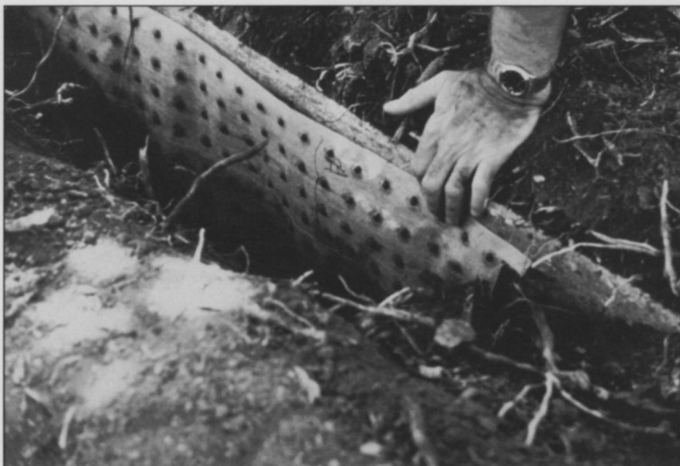
Typar® Bio-barrier® root control fabric is installed between the tree and sidewalk.
