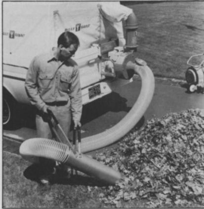
back of a truck. Its powerful vacuum sucks leaves through a 7- or 8-inch diameter intake hose into an impeller with 1/4-inch steel blades. The debris is pulverized into finer pieces before being discharged into the back of the truck, greatly reducing the bulk of the load and maximizing hauling capacity.
