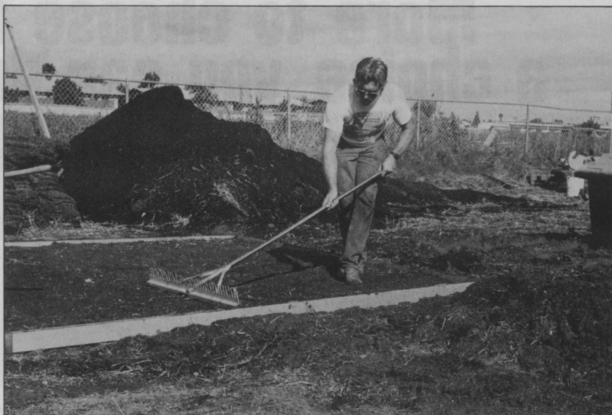
CLT candidate rakes soil mix to level irregularities during the seed and sod portion of CLCA's Certification Test for Landscape Technicians.
