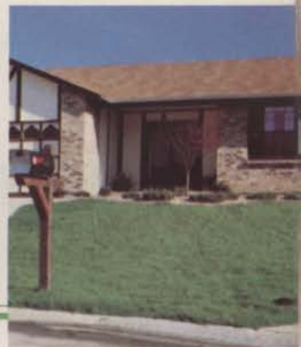
5. COMPLETED RENOVATION DAY 30
