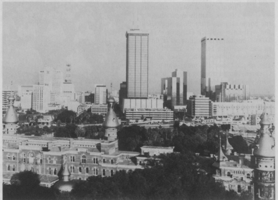
More than $800 million in new construction has dramatically changed downtown Tampa's skyline during the past year. The city is the site of this year's PLCAA annual conference and show.
