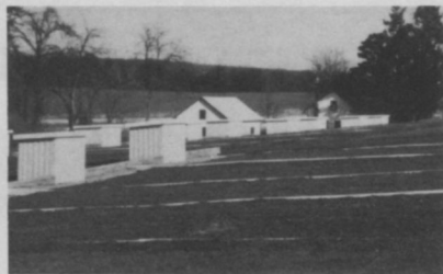
Developing Penn State University runoff research area. The small buildings are built over catch basins at the bottom of the slopes. The facility is designed to monitor water quality after application of nutrients and pesticides.
