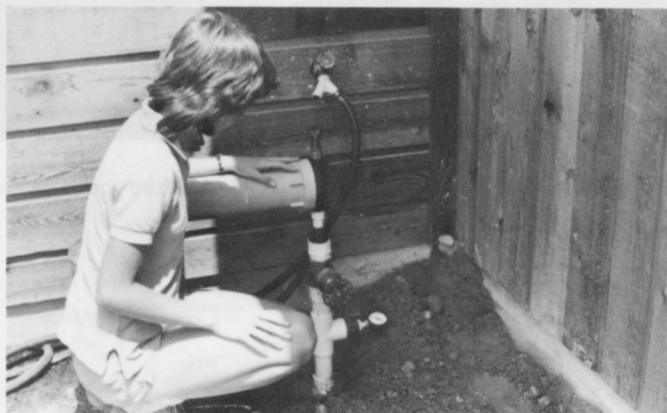
Figure 4. The subsurface watering system can be attached to an outside faucet. A cartridge or screen filter is a basic component of the system.
