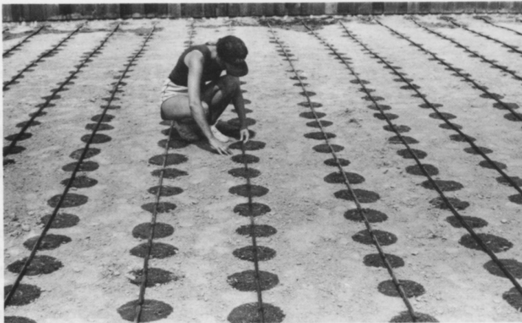
Figure 5. Flush the supply lines before activating the system. Operate the system for a sufficient time to detect faulty connections and to observe wetting patterns.
