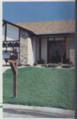
5. COMPLETE RENOVATION DAY 30
