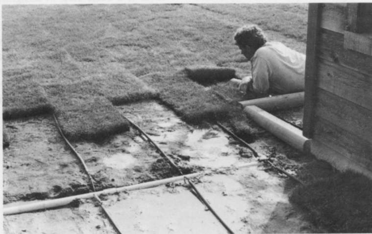
Figure 6. Soil should be thoroughly moistened before sod is placed over drip hose.
