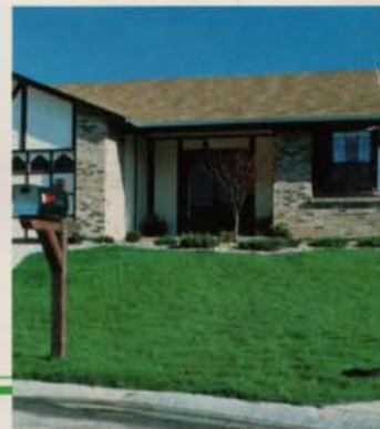
5. COMPLETED RENOVATION DAY 30
