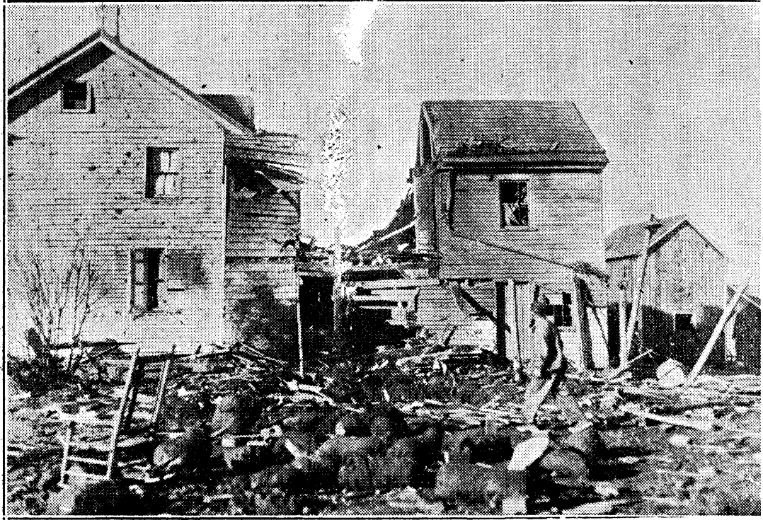
Ripped from its moorings by the terrific explosion of a 10,000-gallon still, a three-ton boiler shot through the walls of Frederick Danner's farmhouse in Woodstown, N. J., narrowly missing its occupants, and killing two men by hurling them 200 feet away. The still was in a barn on Danners' property, which he had leased to the two who were killed.
