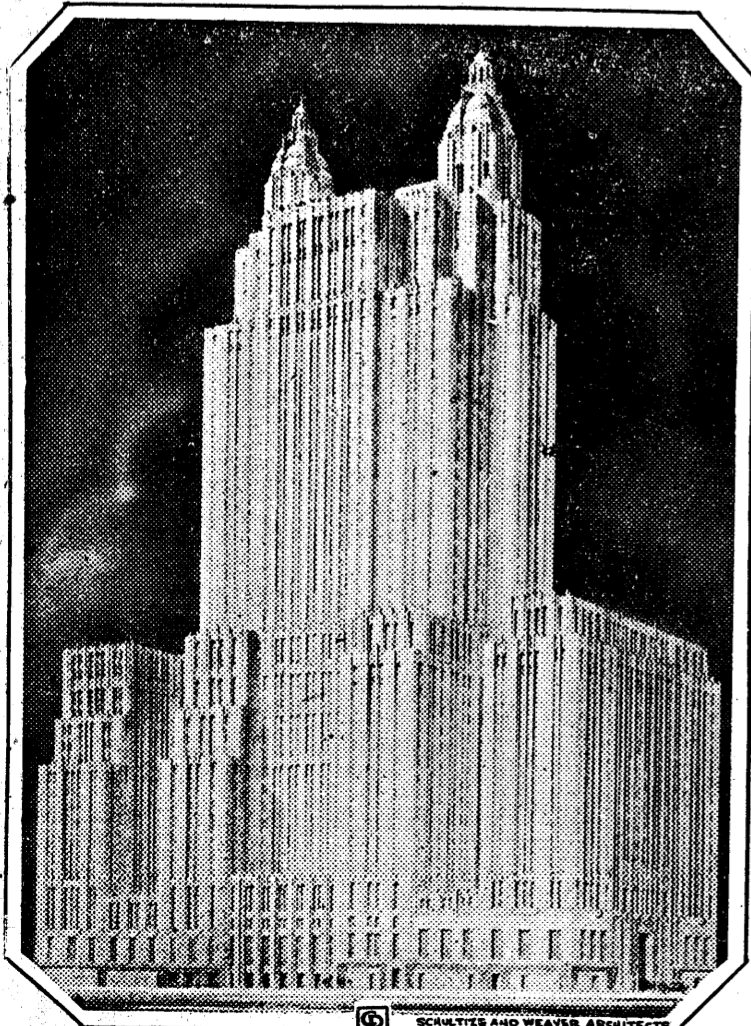
Rising 43 stories in the exclusive section of Park avenue, New York, the new Waldorf-Astoria may be the costliest hotel ever erected. At least the plans call for the expenditure of many millions. Work soon is to begin. There will be 2,200 rooms and a ballroom four stories high.
