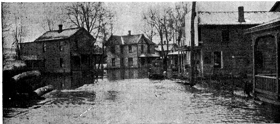
Flood scene in Warren, Pa. Clark street, one block south of business section. As floods threatened to top previous records in parts of Pennsylvania, New York and eastern Ohio, a cold wave checked the rising waters.
