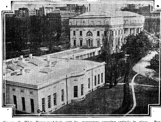
Here is the way the White House roof looks with its temporary covering entirely in place. Beneath this structure a large force of men is rushing repairs, which include steel supports. Contractors found the old roof had long been in danger of crashing. The executive offices are to the left of the picture. They are undisturbed and President Coolidge transacts business in them daily, motoring from the temporary White House in Dupont. The front of the comb, instead of be-
