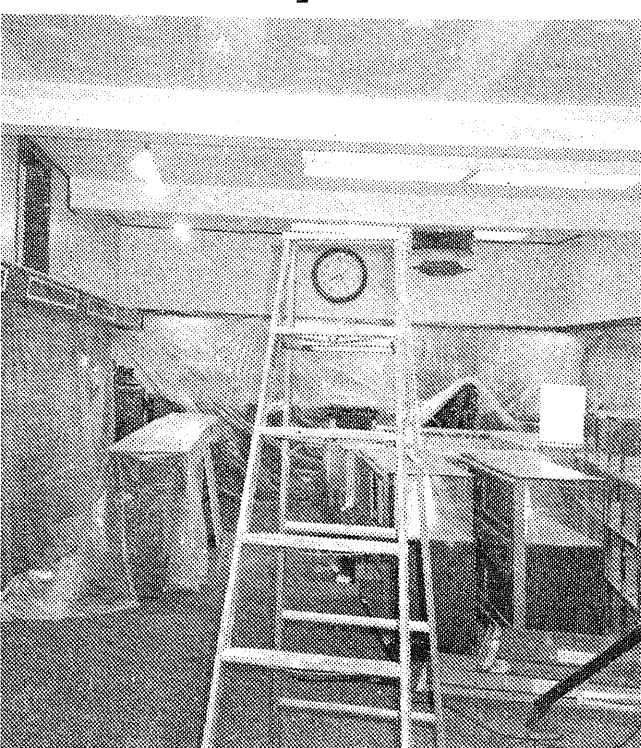
REPAIRS: Layher Jewelers Inc. store in Downtown Sebawaing underwent some major repairs last week, after a broken water pipe in the ceiling decided to shower the showroom. Damage estimates are still being made.
