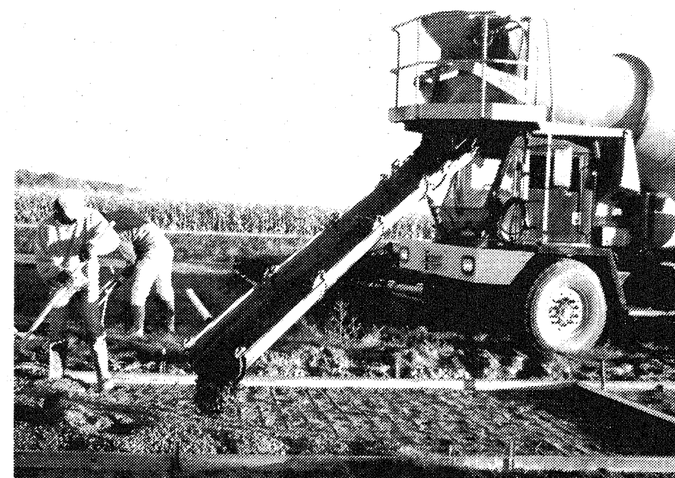
USA SCHOOL WORK: Wolgast Construction Co. is making some real progress on the USA Middle school addition and athletic complex work at the high school complex. Workers are busy with sidewalk that will go to the new athletic complex. The football field has been seeded and the base work for the all-weather track will begin soon. Also, workers expect to have the Middle School wing enclosed by mid November to begin interior work. Completion of the addition is expected in February. MARY DRIER PHOTO
