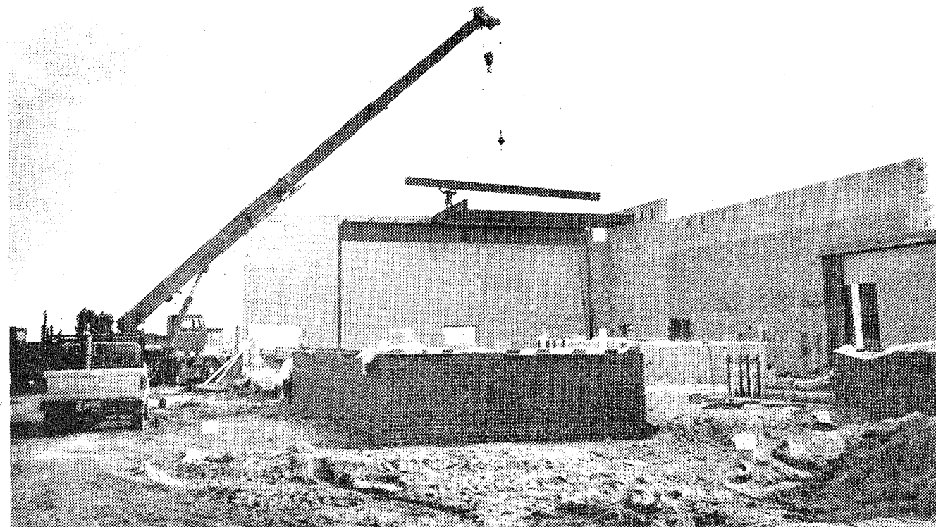
CASEVILLE SCHOOL CONSTRUCTION was underway last December, when this girder-raising shot was taken...
