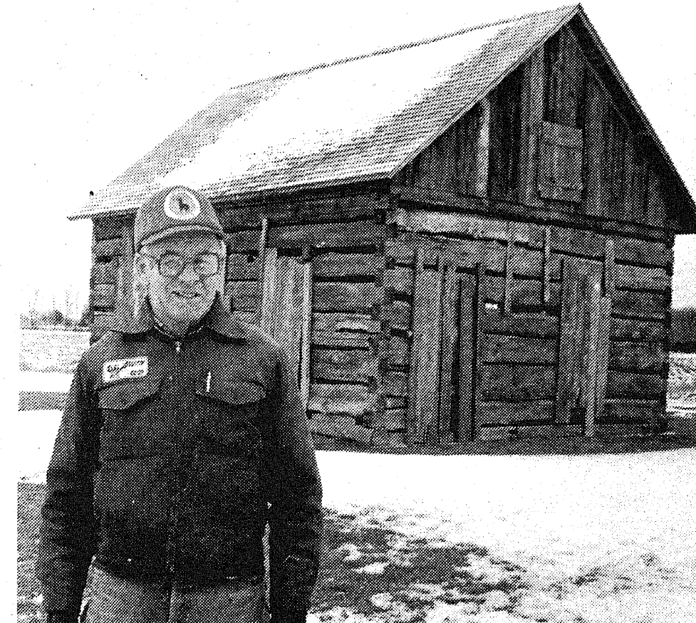
HISTORIC CABIN: Elkton Historical Society President Leonard Bumhoffer poses with the nearly finished log cabin moved to Ackerman Memorial Park last summer. The historic structure was donated by Mr. and Mrs. Henry Schoenhals of Port Austin. The public is invited to an Historical Society meeting at Elkton Village Hall at 7 p.m. on Tuesday, Jan. 27 and other monthly meetings slated for the fourth Tuesday of each month.
