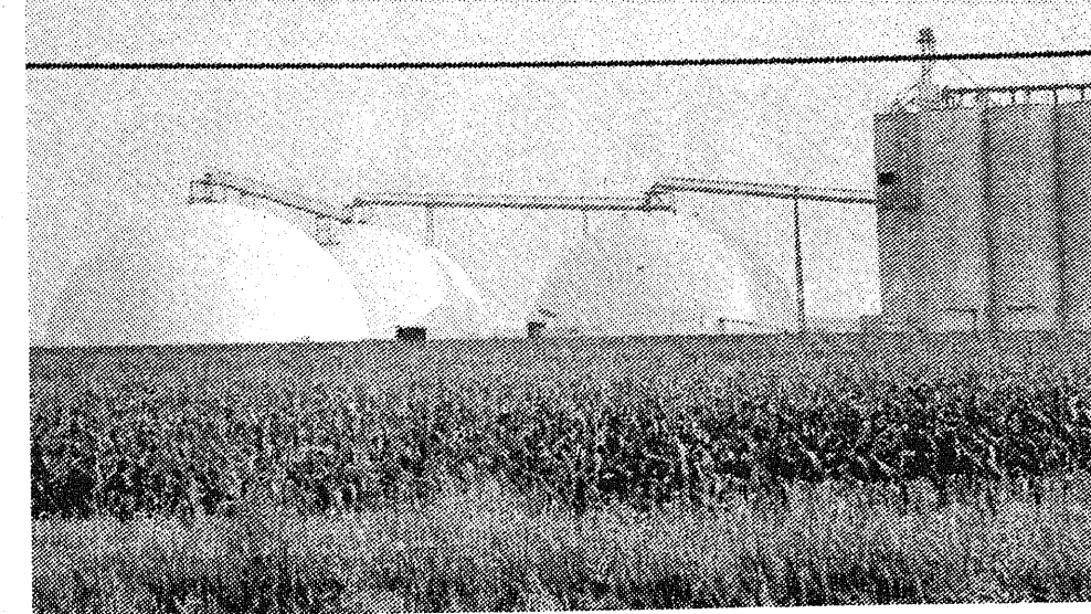
DOMES COMPLETE: The third and final covered dome is being readied for servicing this fall's grain crop at the Elkton Plant of Co-operative Elevator Company, on M-142 east of Elkton. The elevator "legs" linking the domes to existing concrete silos are also installed, as the photo shows.
