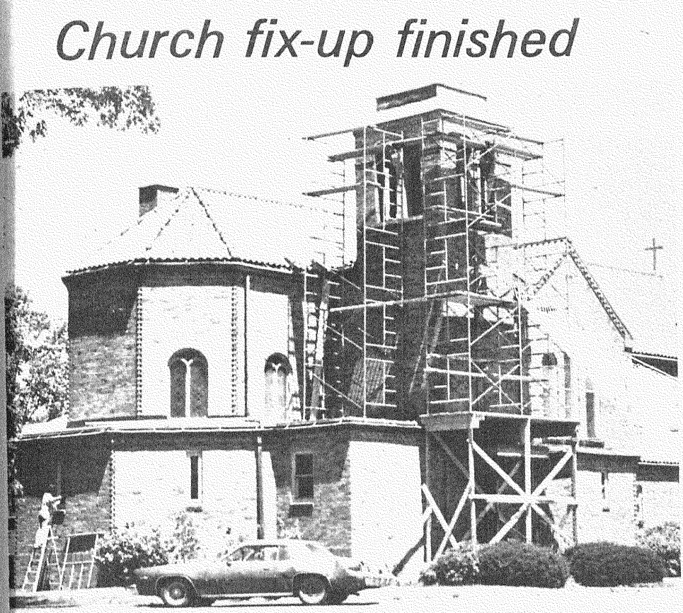
WORK HAS BEEN COMPLETED ON THE tower of St. Francis Borgia Catholic Church in Pigeon and it's now "picture perfect," as shown above. Workmen were busy replacing bricks on the structure, both inside and out. PHOTO BY RICH SWARTZENDORBER
