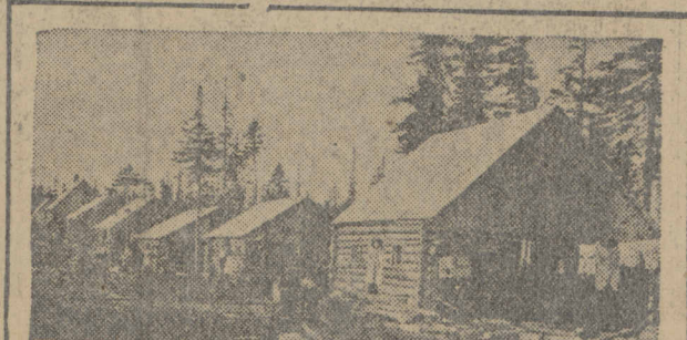
Milwaukee Avenue, a street in Shelter Bay. Houses built by the French Canadian workmen from trees cut down within a few yards of their home sites. The Tribune is now building a church and school for the benefit of its employees, and will assist them in erecting a better type of house.
