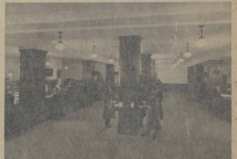
NEW PUBLIC SERVICE QUARTERS
