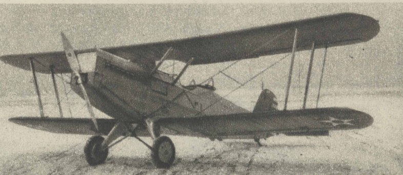
A Douglas observation plane, model for the first commercial Douglas, the DC-1, also in scale to the DC-4. It was approximately 32 feet long and carried two persons and mail or baggage.
