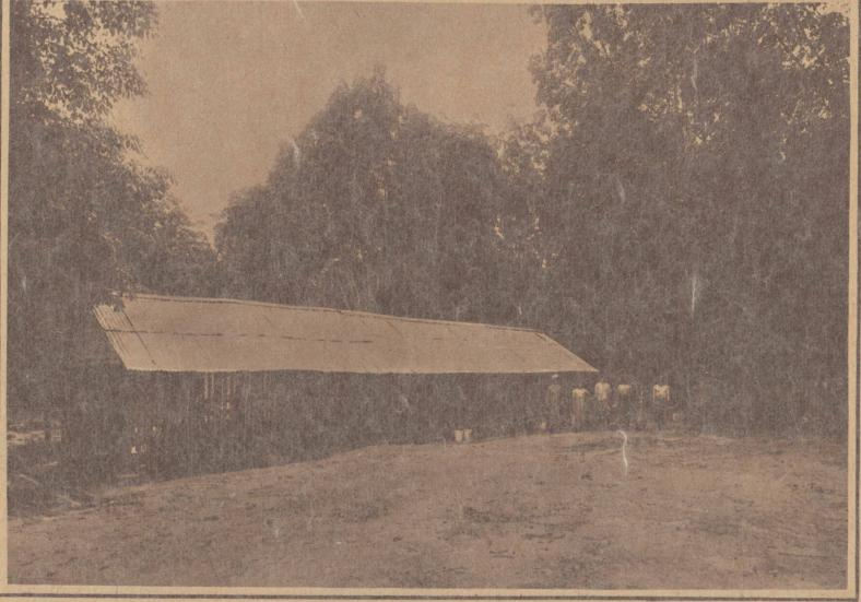
THE TREATING SHED is the first destination of the rubber sap. Here the latex is coagulated with acid in large vats, thoroughly washed to remove all trace of acid, and then rolled into sheets, rolled and rerolled to remove as much water as possible.
