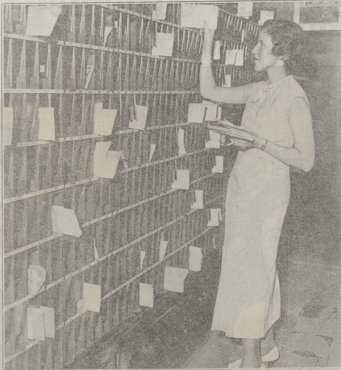
(Photos courtesy Bismarck hotel, Chicago.) When letter is inserted the metal flap is pushed back. This causes green light to flash in guest's room.
