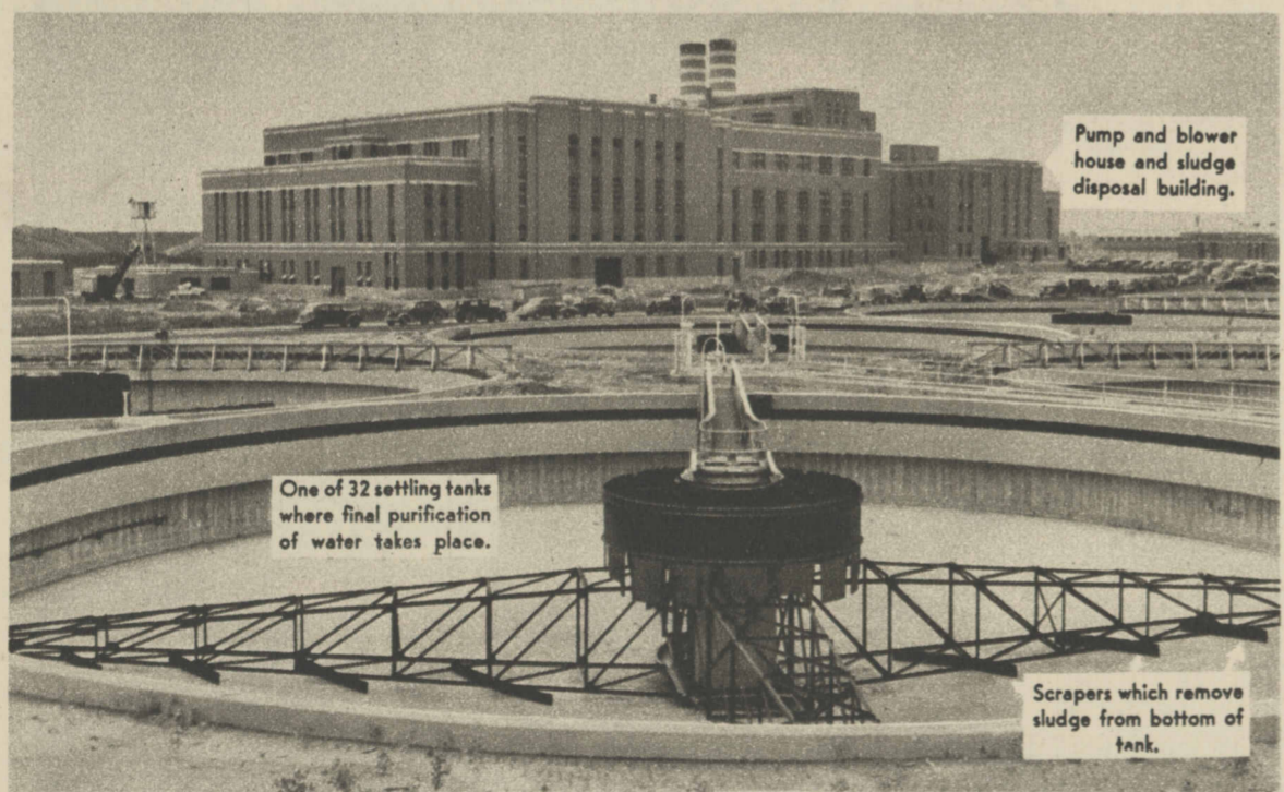
General view of southwest sewage treatment works, capable of handling 600,000,000 gallons of sewage a day.
