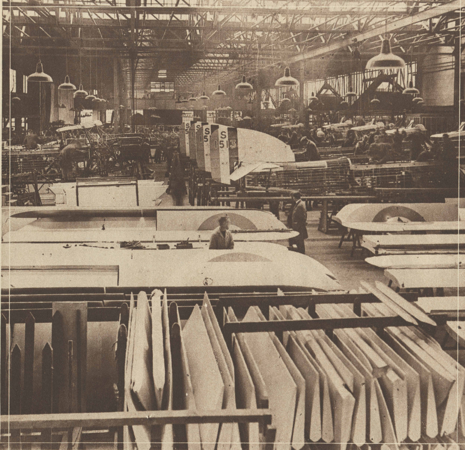
CREATION OF AN AIR FORCE—Scenes in a great airplane factory at Hayes, Middlesex, where fast fighting machines are turned out for the British empire. Above, a general view of ships under construction in the erecting room. (© Acme photo.)
