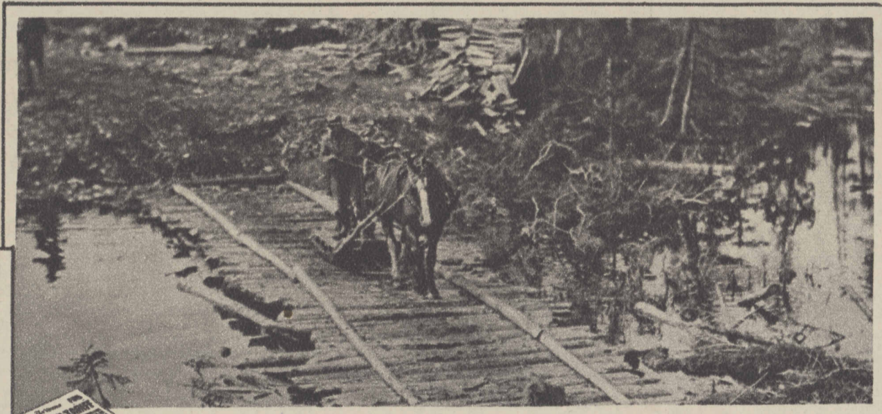
MACADAMLESS ROADS AND SNOWLESS SLEIGHING —Timberland roads are carried across swampy ground by laying a roadbed of logs. This is the type of road known as the "corduroy." The vehicle shown is a "bacognale," a crude sleigh used extensively, even when the snow has gone, for hauling supplies over rough forest trails.
