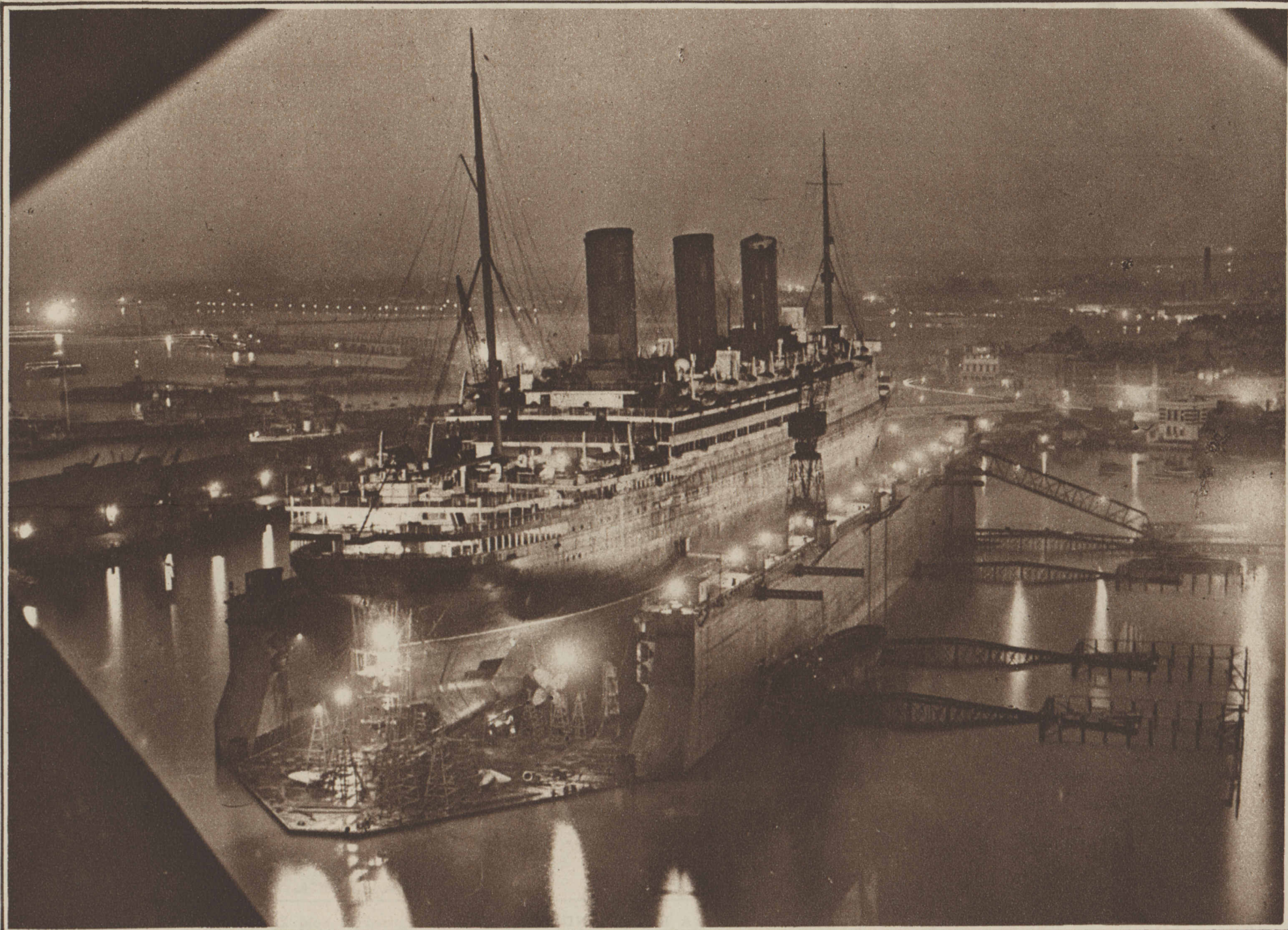
NIGHTFALL—Illuminated by a flood of lights, the Berengaria is seen in her Southampton dry dock, where overhauling crews labor night and day in the refurbishing of the huge liner. (Associated Press photo.)
